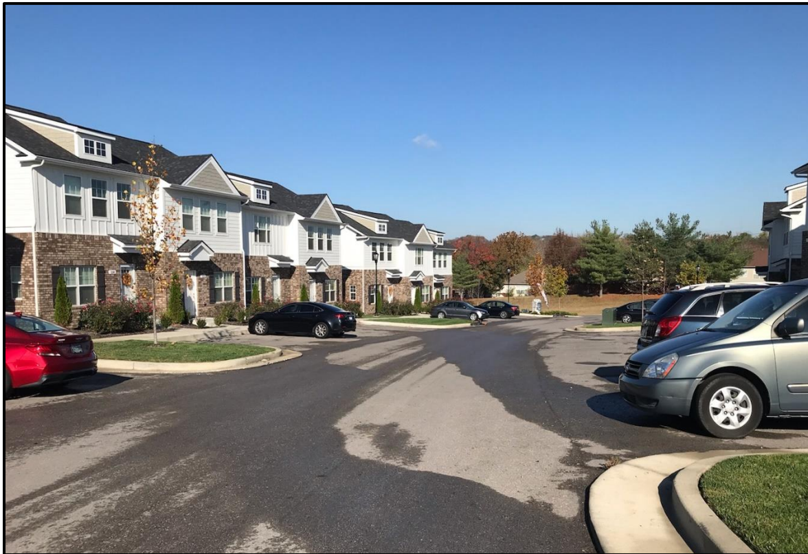
Photo: Dry Creek Commons Phase One – November 1, 2022
